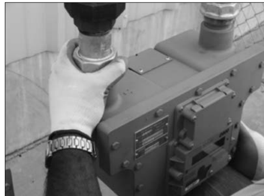
Figure 5.2 - Connect meter ferrule into swivel nut on the gas supply side
