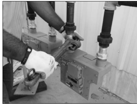
Figure 5.5 - Use a pipe wrench to tighten swivel nuts.
